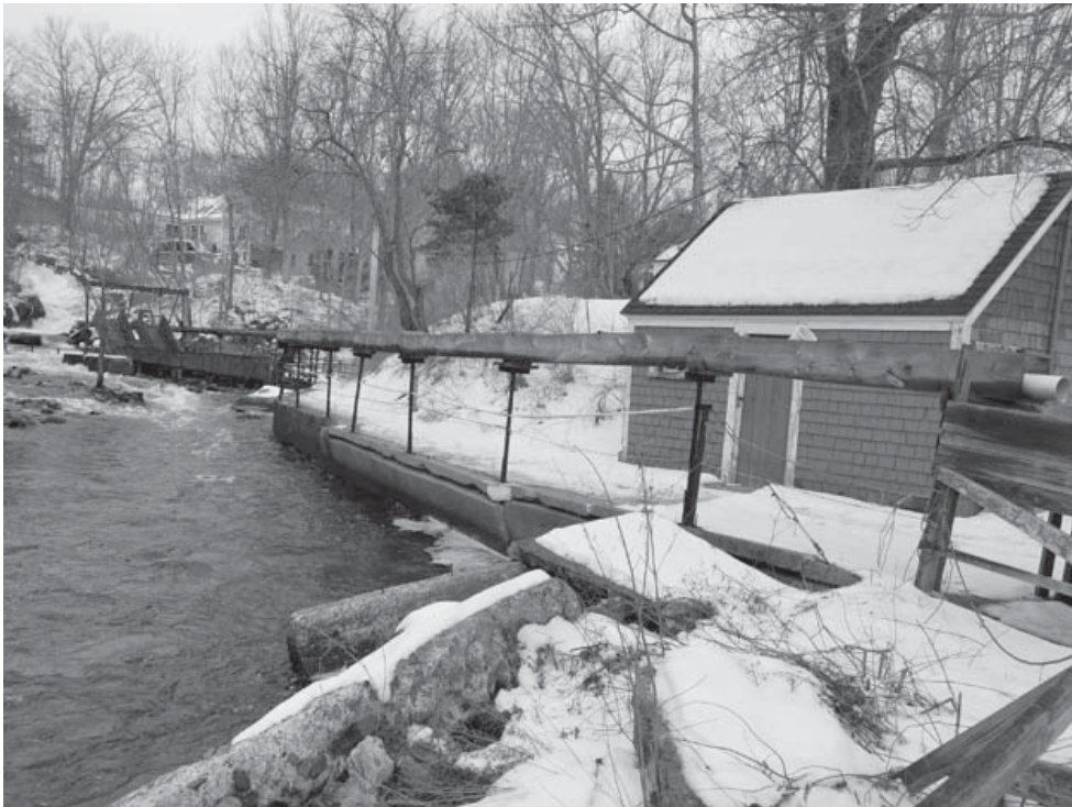
The rebuilt wooden trough that aids in harvesting the alewives.
