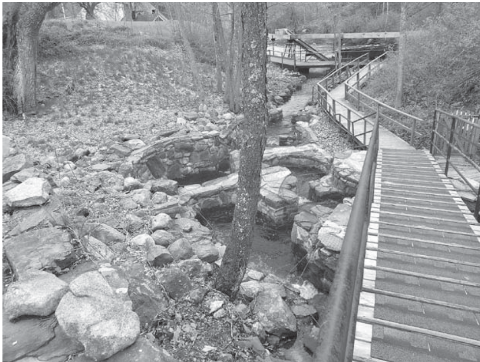
Completed restoration by the footbridge, 2016. (Russ Williams photo)
