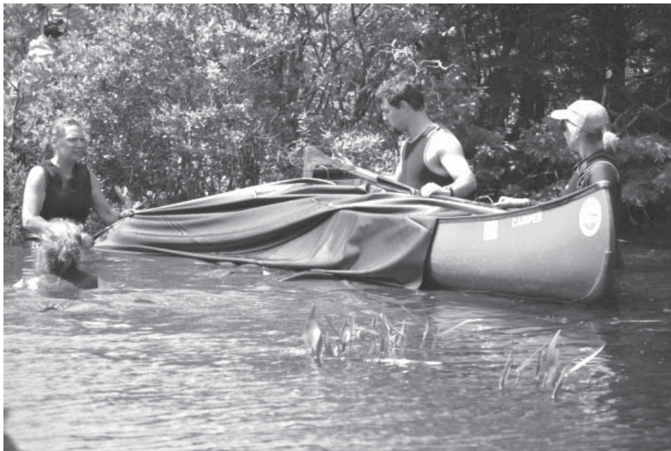
Garrison Beck, DLWA Senior Program Manager, and members from the DEP installing the pond liner.
