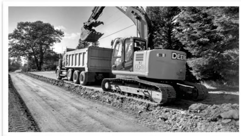
Therault Construction reconstructing part of East Road – summer of 2015
