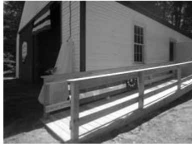
Handicap accessible ramp at Razorville Hall
