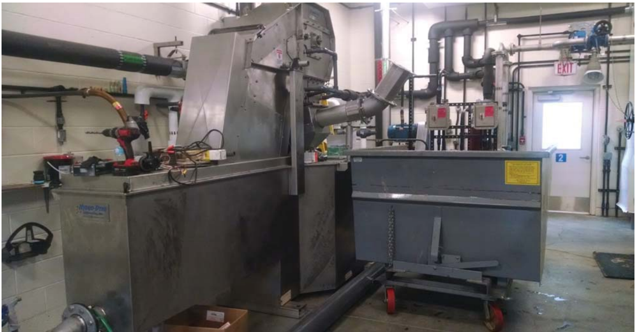
New Septage Screening Equipment
