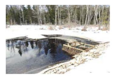
The beaver deceiver that was installed to prevent the beavers from obstructing the culvert and causing flooding of the north entrance road to the park.
