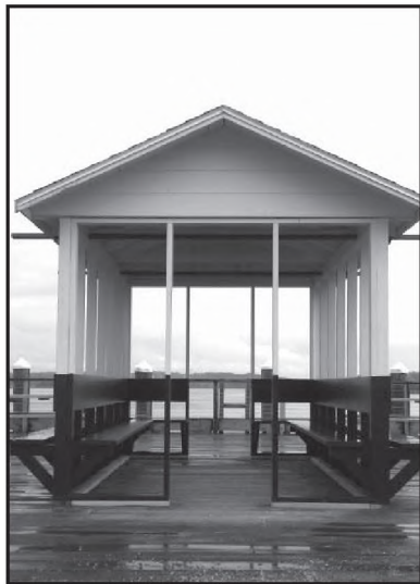
Newly re-constructed Town Dock Gazebo by Public Works, Henry Erhard
