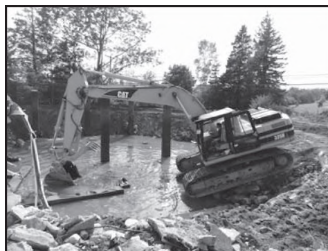
CCLP under construction
