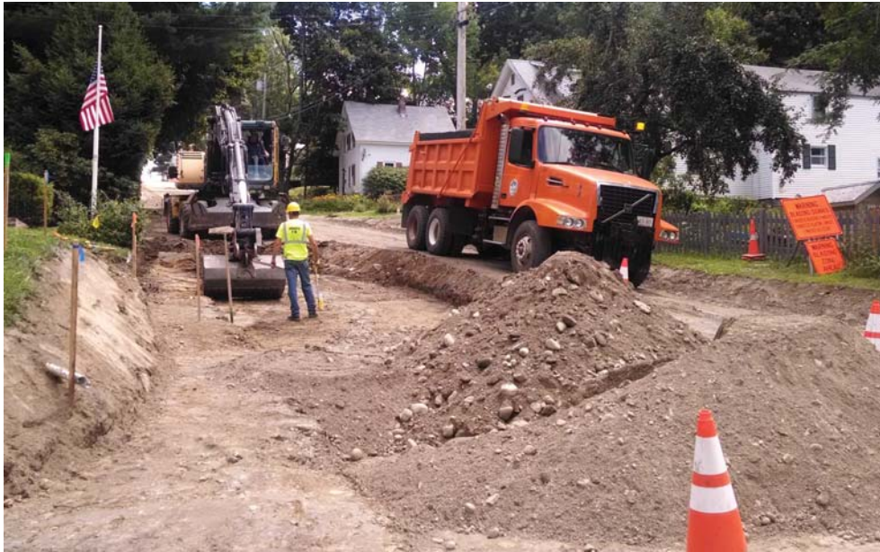
School Street Construction during the summer of 2015.
