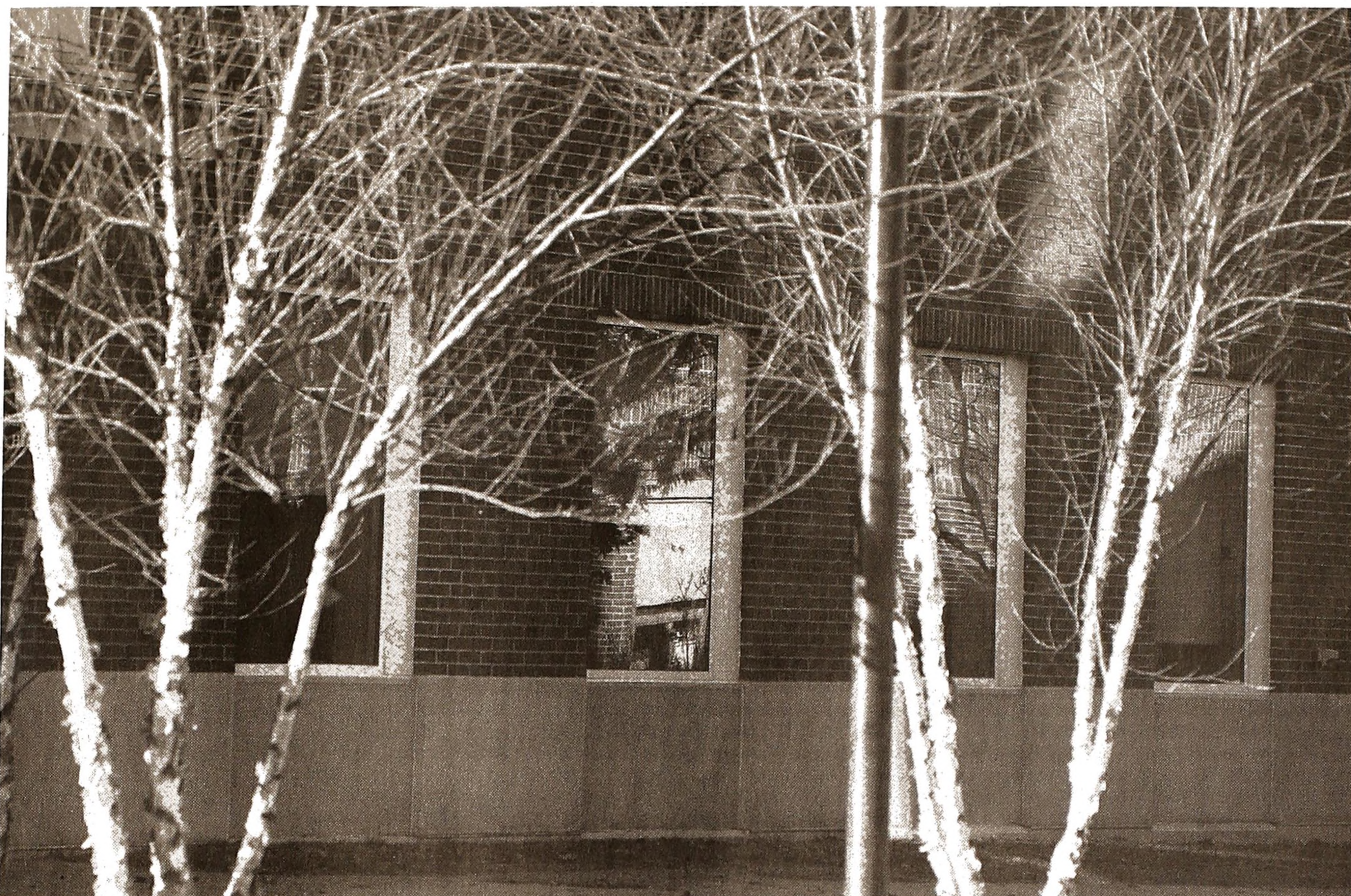
First floor of Barrows Hall from the outside
