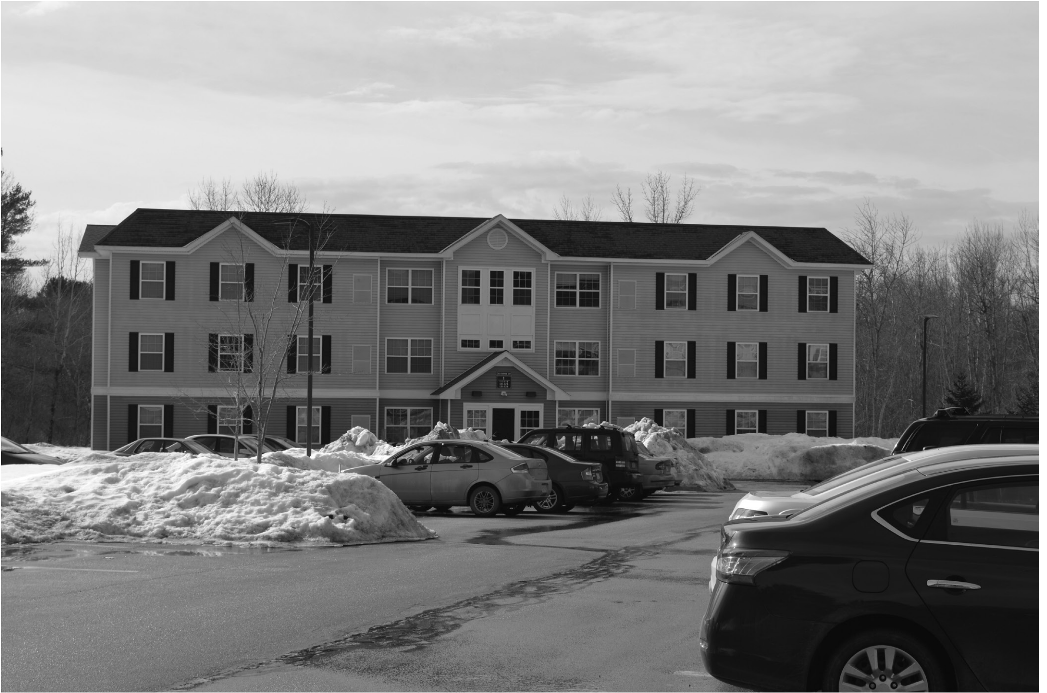
Apartment buildings at Orchard Trails (OT) in Orono.
