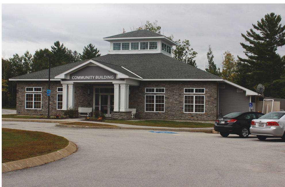
The Community Building at Orchard Trails.
