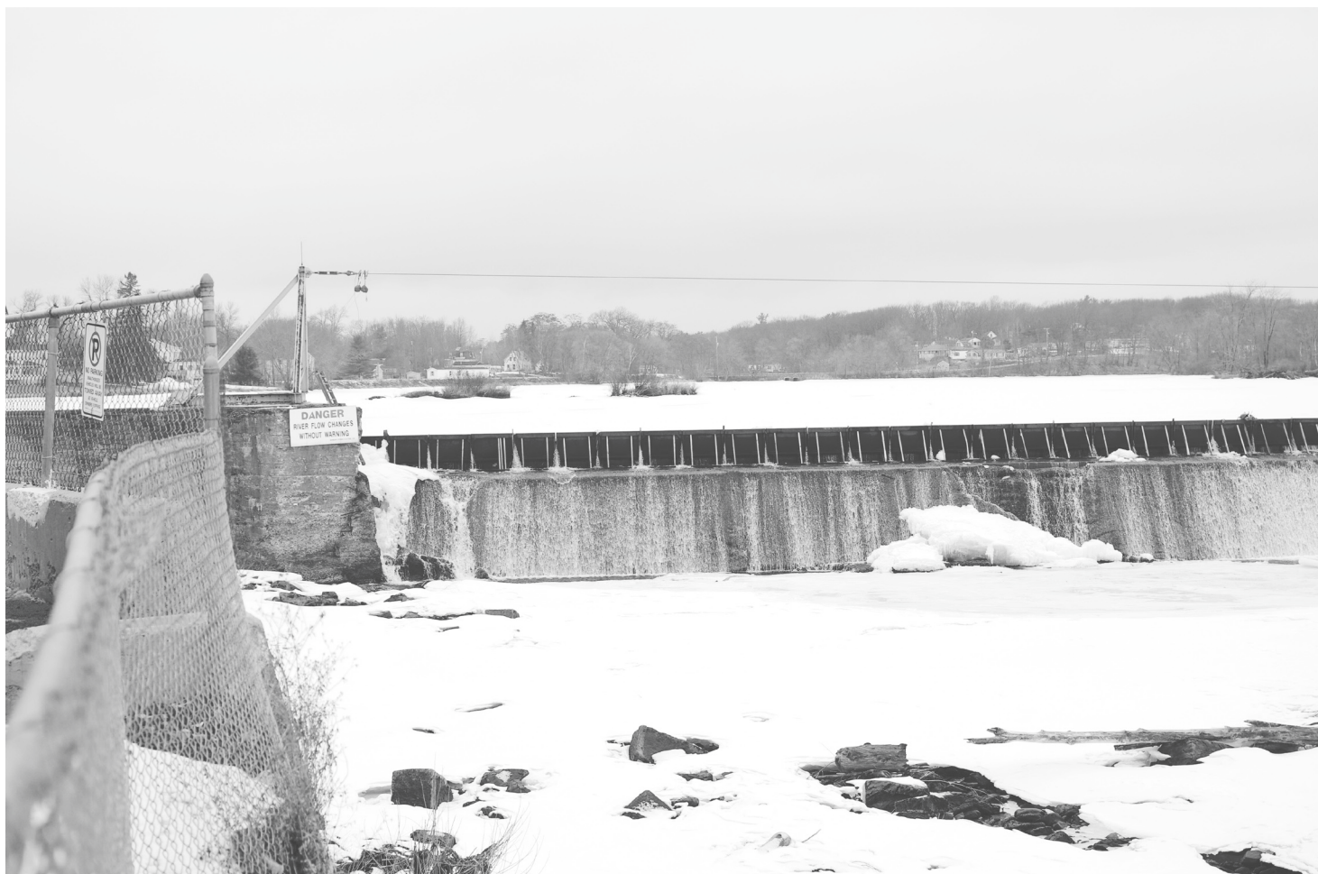
A male Black Bear Hydro Partners employee was taken to Eastern Maine Medical Center in Bangor on Wednesday morning after becoming trapped under a splash board on this dam spanning the Penobscot River. He suffered a leg injury and hypothermia.
