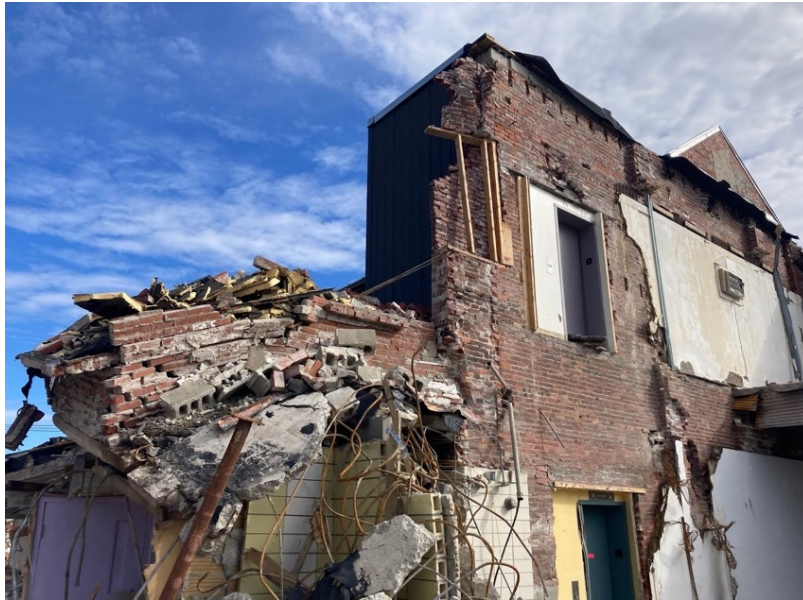
Figure 59: “Site-Work, horizon line of elevator used for light-work with glass; completely altered.”
