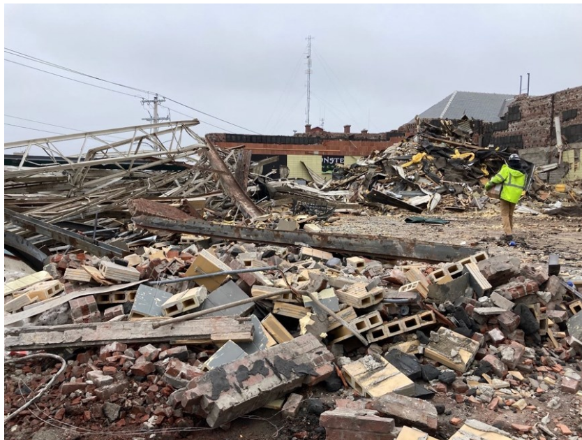
Figure 36: “Site-Work: Alloy Group at work.” March 2024
