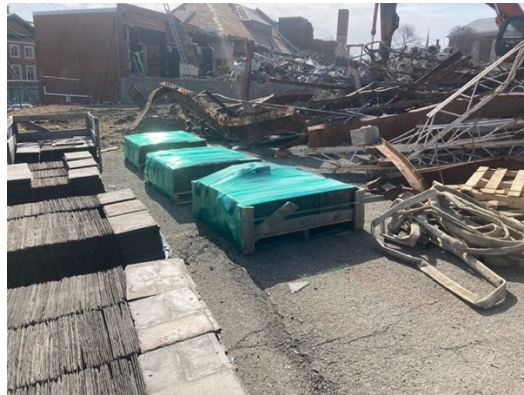
Figure 71: “Green saran wrap covers rescued slate.” March 2024.
