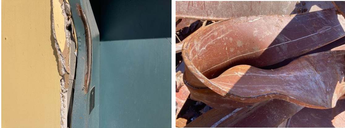
Figure 121. “Site-Work, observation of material 1.” Figure 122. “Site-Work, observation of material 2.”
