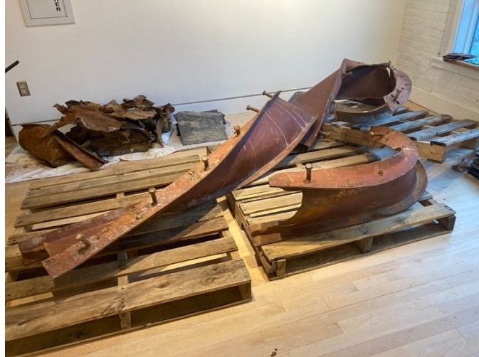
Figure 117. "Site-work, repositioning I-beam onto pallets sourced from 127 Hammond St"
