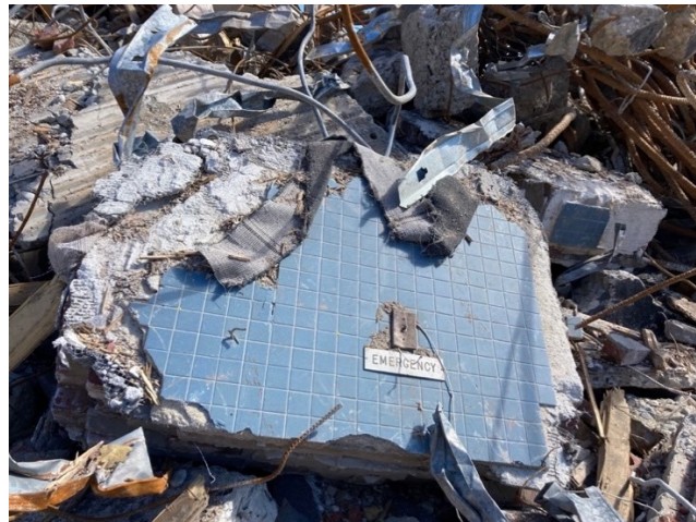
Figure 64: “Site-Work, pool wall lays horizontal.” April 2024
