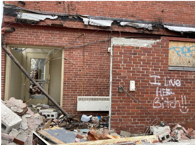
Figure 32: “Front façade altered by demolition. February 2024.”
