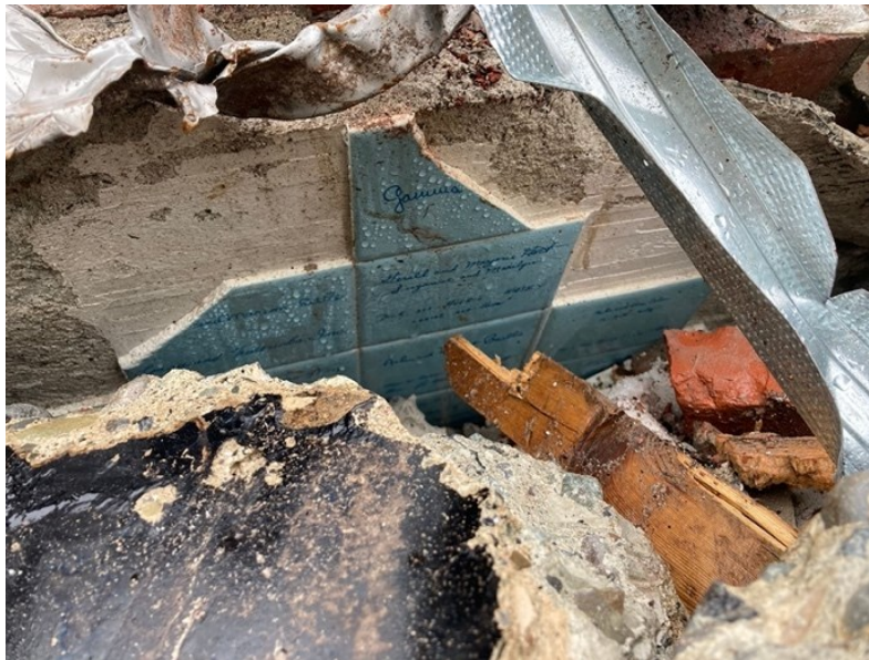
Figure 60: “Site-Work, YMCA Builders Wall encountered, now rubble.” March 2024.
