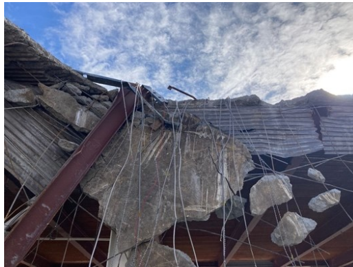
Figure 19: “Site-Work, documenting demolition, observing patterns.” April 2024.
