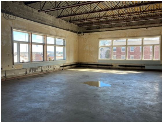
Figure 15: “Site-Work, reflections 1. 3 rd Floor”
