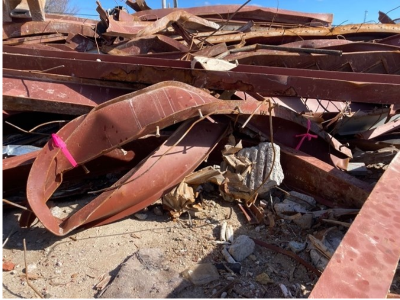
Figure 75: “Site-Work, pink flagging around I-beams in anticipation of exposition.” May 2024
