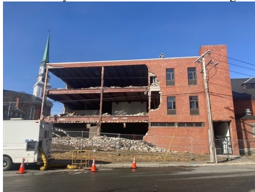
Figure 46: “Deconstruction along Hammond and Court St.” April 2024
