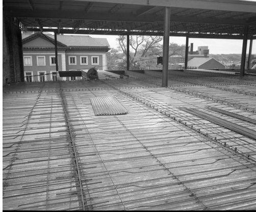
Figure 39: “Bangor Public Library. 1969-1973 Building YMCA. Corrugated tin visible.”
