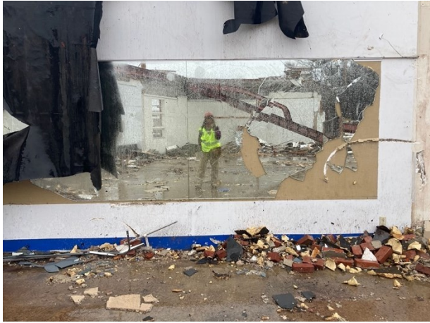
Figure 24: "Site-Work Selfie. March 28 th 2024."
