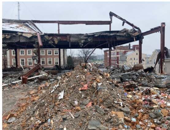
Figure 40: “Exposed corrugated tin from 1979 now visible in 2024.”
