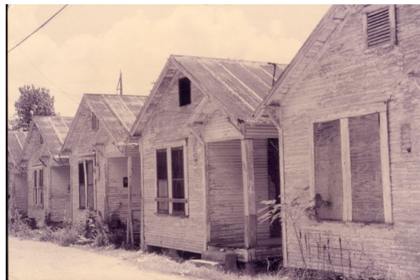
Figure 47: “Rowe House Before Renovation. Photo: Sheryl Tucker of Project Rowe Houses.”
