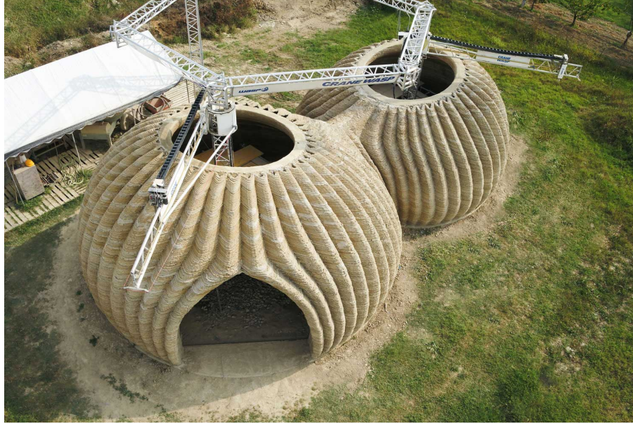
Figure 2.7: Tecla house printed with earthen materials by WASP [6]
