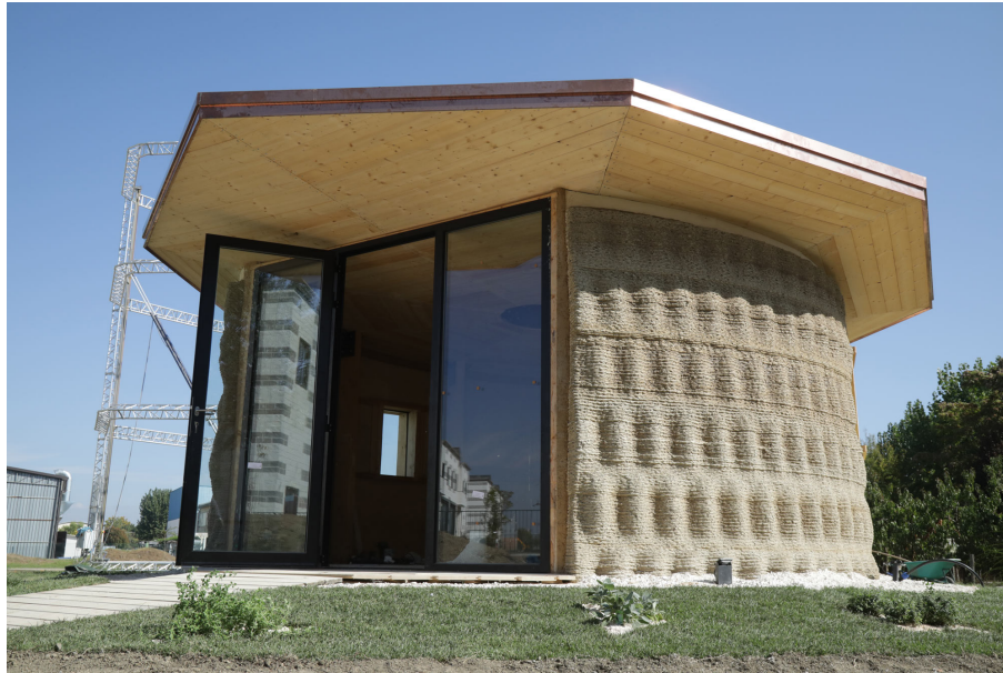
Figure 2.6: Gaia house printed with earthen materials by WASP [5]
