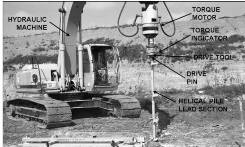
Figure 2.29. Helical anchor installation (Perko 2009).
