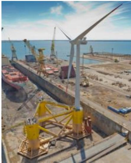
Figure 1.4. 2-MW WindFloat quayside (Principle, 2014)
