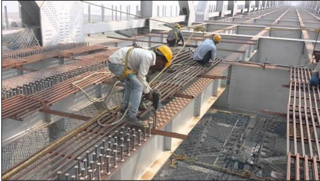
Figure 67: Drawn Arc Stud Welding [54]
