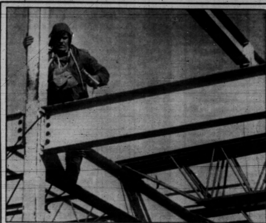
Joe Legery of Old Town takes a minute to look over the work being done on the Surface Science and Environmental Chemistry Building.
