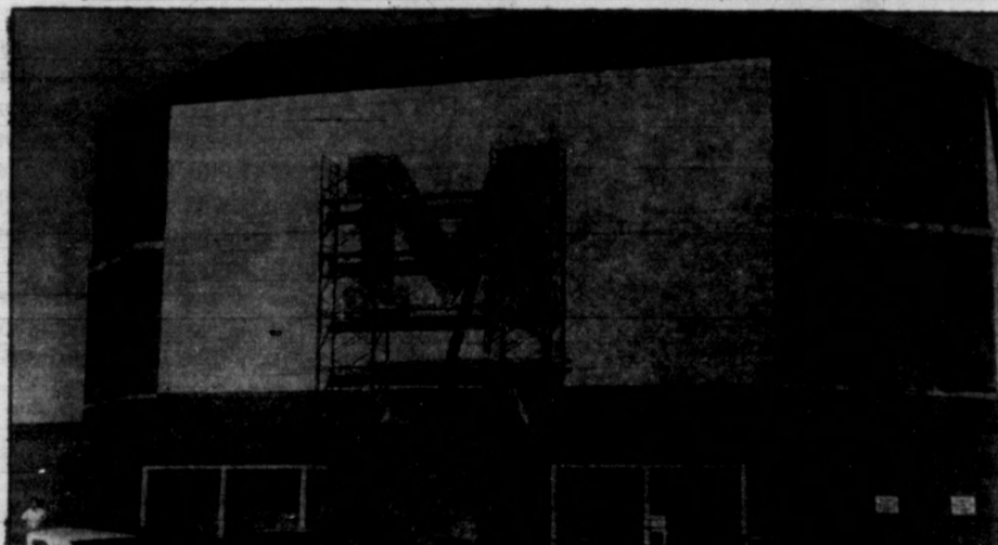
The Memorial Gym is currently undergoing interior construction of office space and handicap facilities. (Campus photo)
