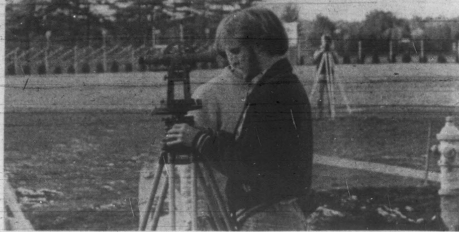
At Mahaney Diamond this week, work began on new bleachers, which will include 500 permanent seats.
