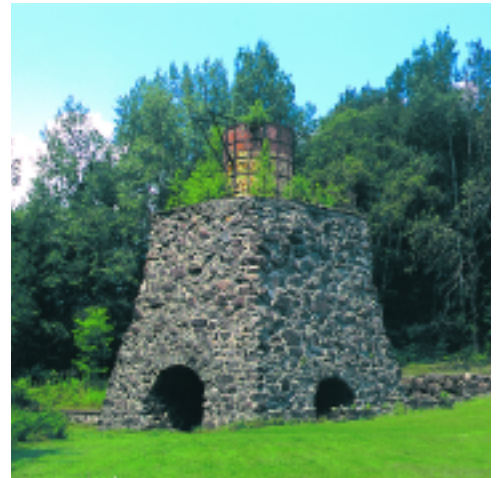
Katahdin Iron Works A restored stone blast furnace and charcoal kiln on the site of a 19th century iron works that produced 18-20 tons of raw iron daily during its periods of peak operation in the 1880s.
