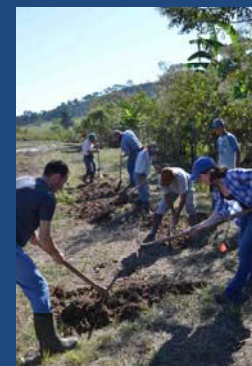
LEFT: Digging an upstream swale.
