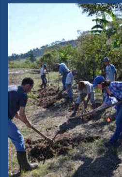
LEFT: Digging an upstream swale.
