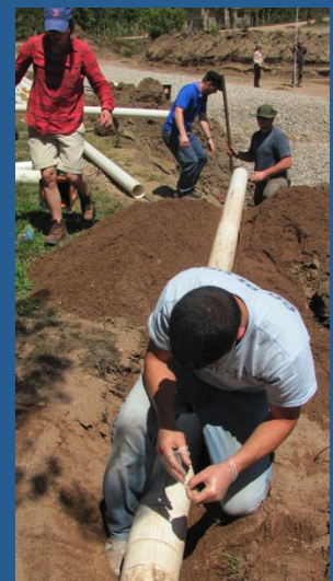
Daniel Gerges gluing pipe together during the recent trip to Dulce Vivir.
