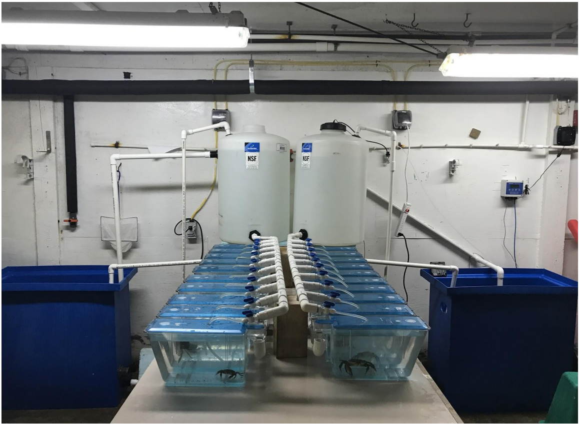
Figure 2. Completed ALCOAST during Trial 1. The acidified system is on the right and the control system is on the left.
