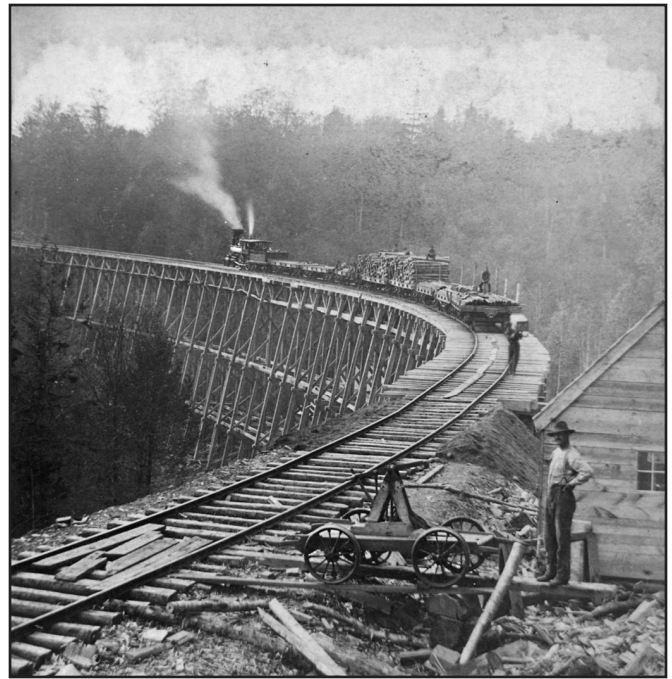
In 1883 the B&A finished the Bunker Brook Trestle and completed the rail line up the valley from Milo Junction to East Shirley Mills. Most trains, like this one, carried birch to the Piscataquis River valley mills. (Charles L. Marston, photographer (1883–1884), courtesy of the Maine Historical Preservation Commission, Augusta, Maine (MHPC.S.4518))
