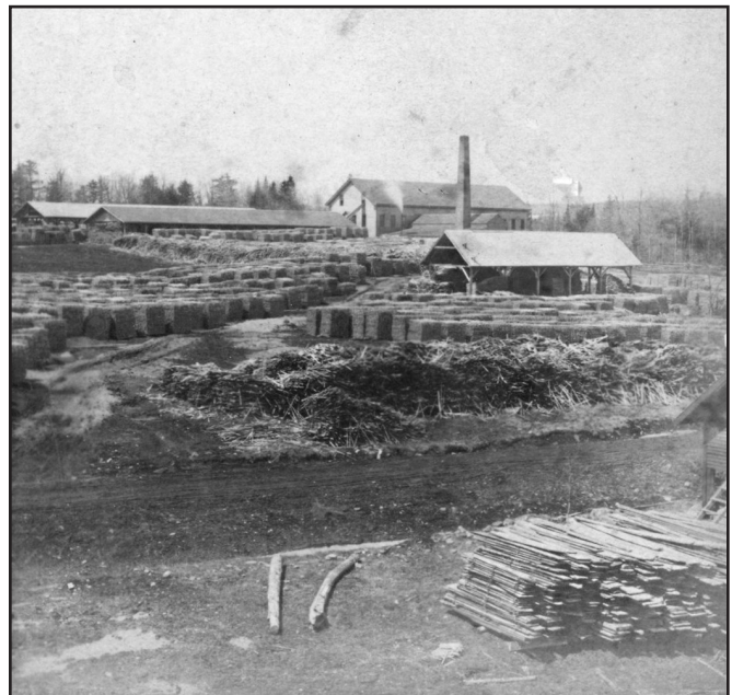
In order to produce 82 spools per minute in 1880, it was not uncommon to see 2,000 cords of birch and 4 million board feet of stacked birch bars at the Dwelley birch mill (1873–1946) at Foxcroft village; it was the largest in the river valley. (unknown photographer (1873–1883), courtesy of the Maine Historical Preservation Commission, Augusta, Maine (MHPC.S.18361))
