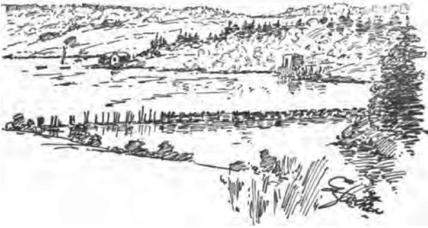
OLD DAM, McCAFFREY'S CREEK
