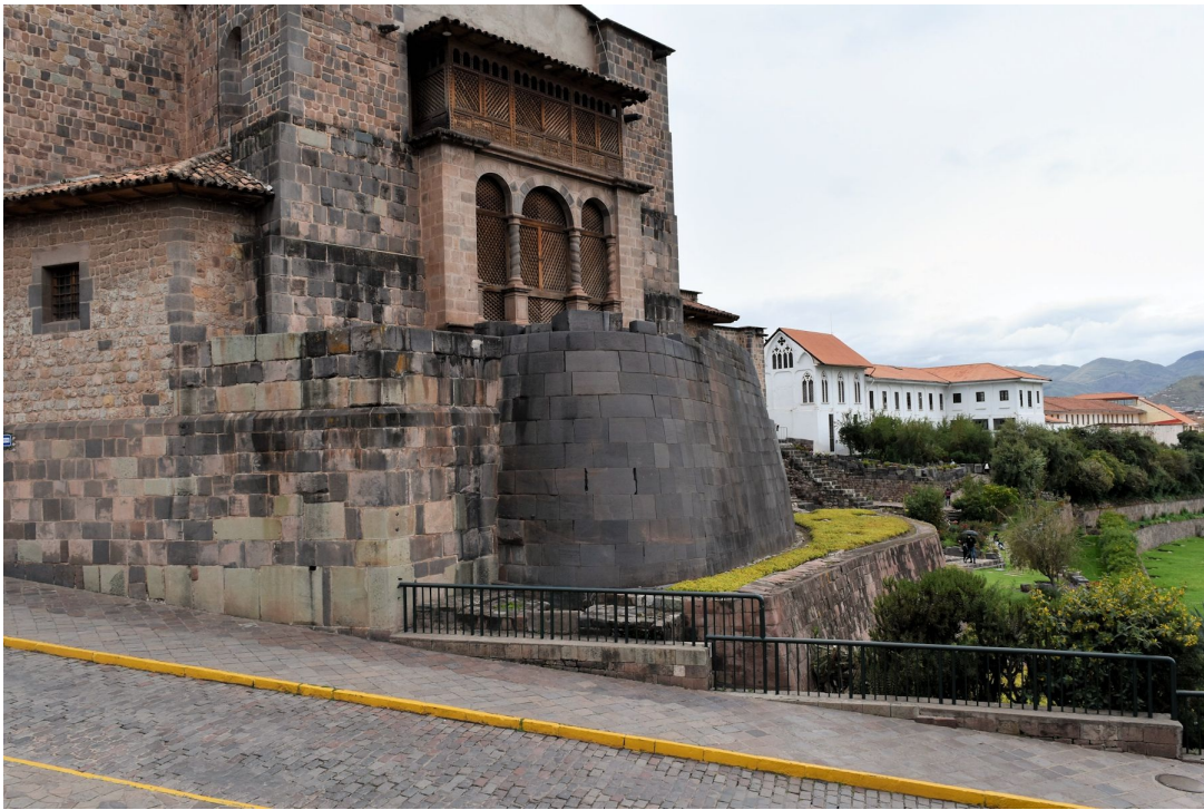
Figure 17. The curved andesite wall of the Qoricancha stands on a stone terrace made of pink andesite. The colonial walls reused diorite blocks.
