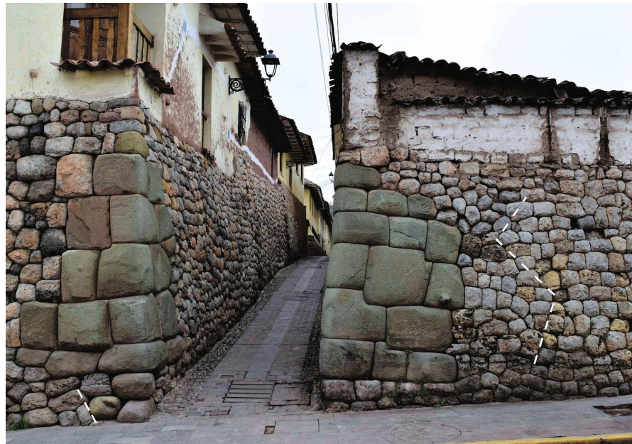
Figure 12. Green diorite wall over a sandstone wall. The dotted lines indicate how the original terrace was cut in order to open the street.
