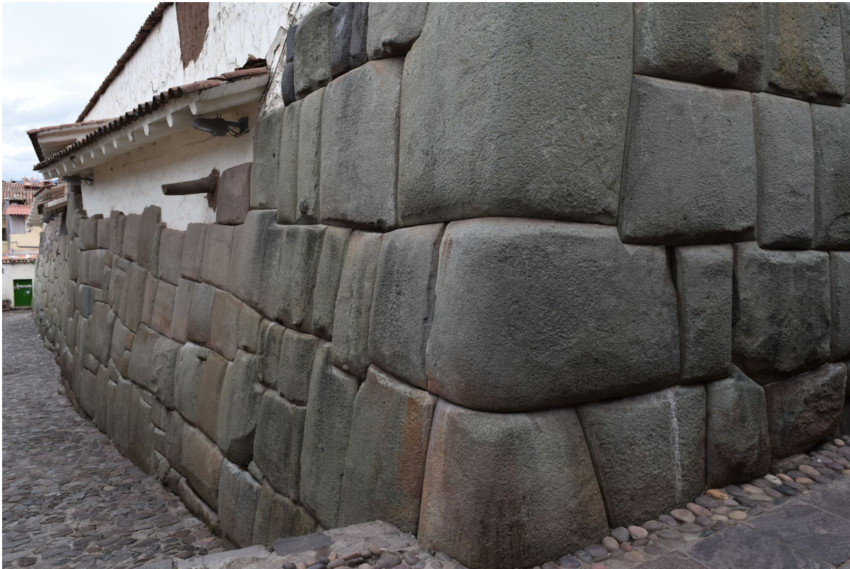
Figure 11. The palace of Inca Roca (Hatunrumiyoc) was constructed with blocks of green diorite.
