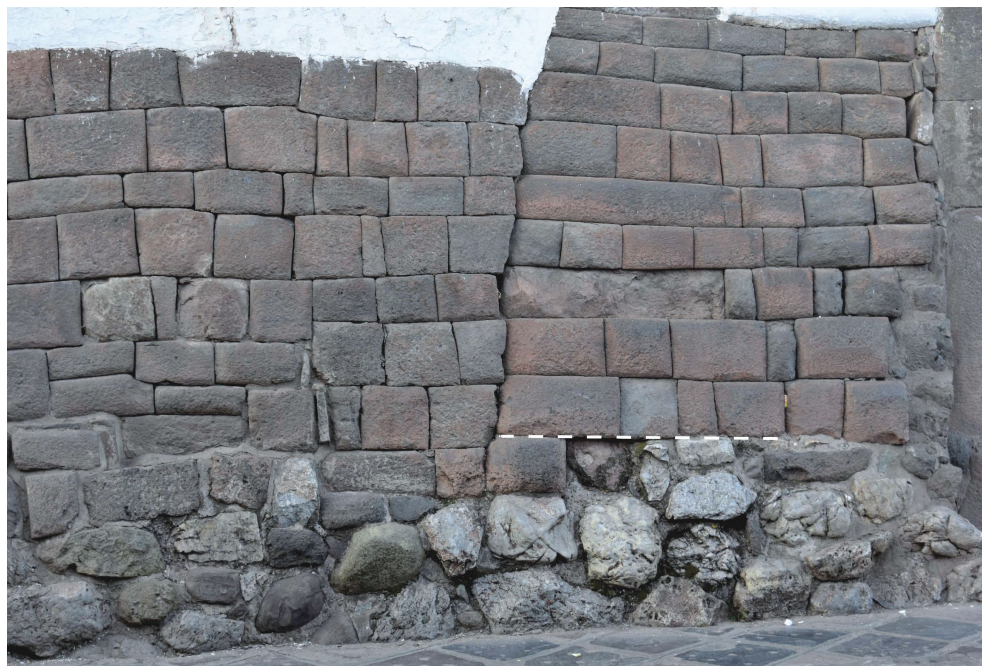
Figure 5. View of the corner of an Inca street that bisected Pampa del Castillo Street. To the viewer's right is a Transitional wall. Below the dotted line is the wall's foundation.
