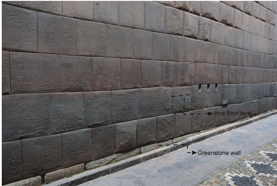
Figure 19. Inca andesite wall on Awaq̄pinta Street. Note the green diorite foundation, the original foundation of the Qoricancha, above the andesite wall. Present day street level is below the Inca street level.
