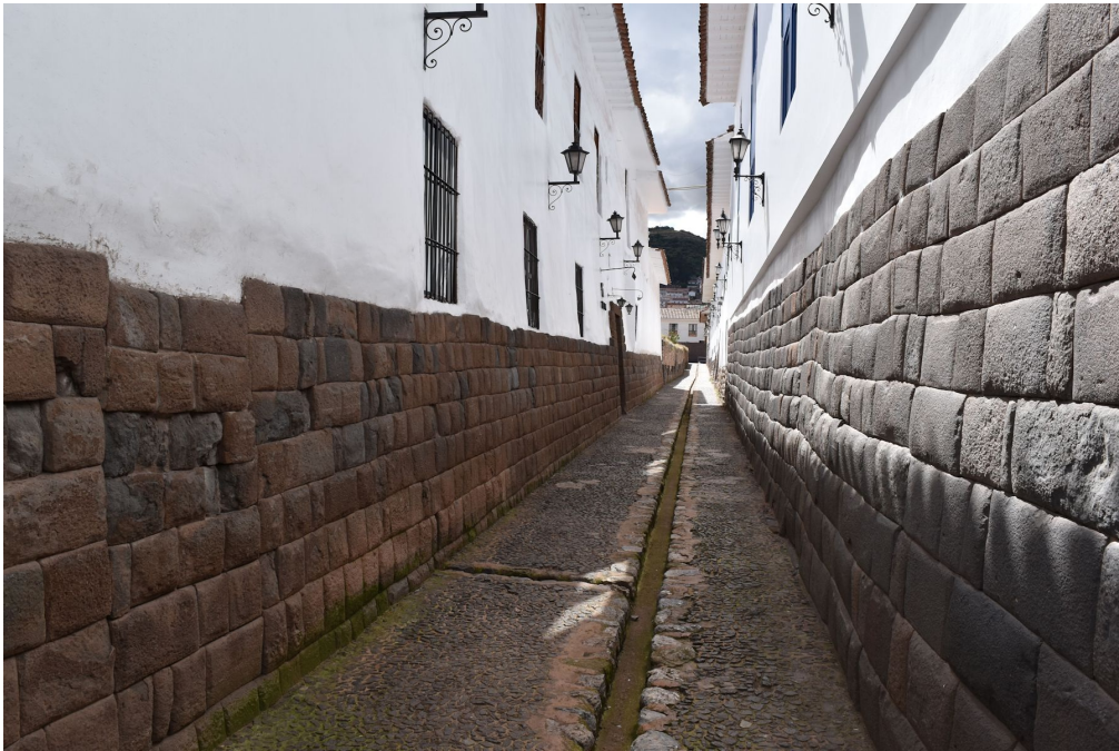
Figure 14. View of Romeritos Street.
