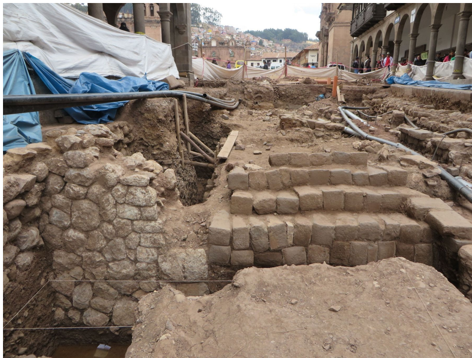
Figure 32. Limestone Inca wall cut by the colonial structure made from reused andesite blocks.
