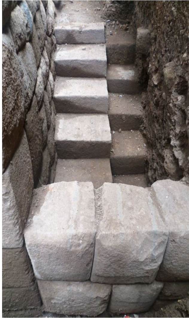
Figure 30. Detail of the blockage of the right stairway with andesite ashlars.
