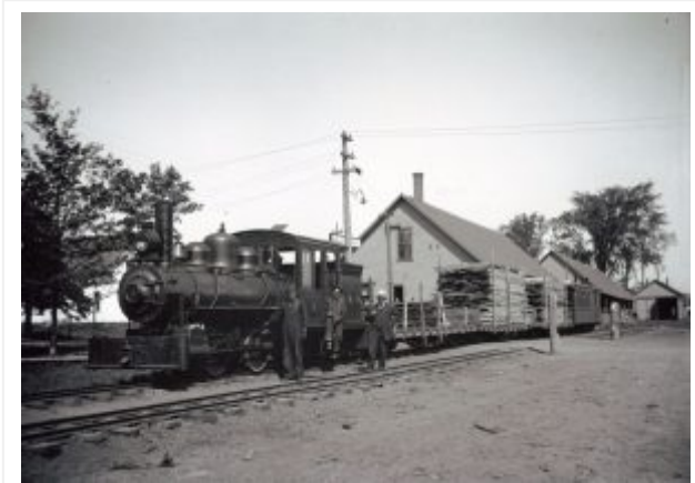
Narrow Gauge Railroad
