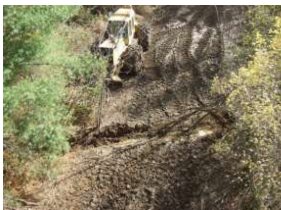
Fig. 2: Completed water bar.
