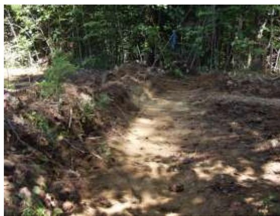
*Fig. 3: Another completed water bar.*
