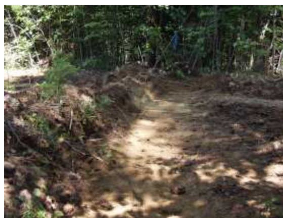
Fig. 3: Another completed water bar.
