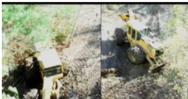
*Fig. 1: Skidder installing water bar. Left, facing downslope. Right, facing upslope. Note skidder's rear tires remain on trail.*
