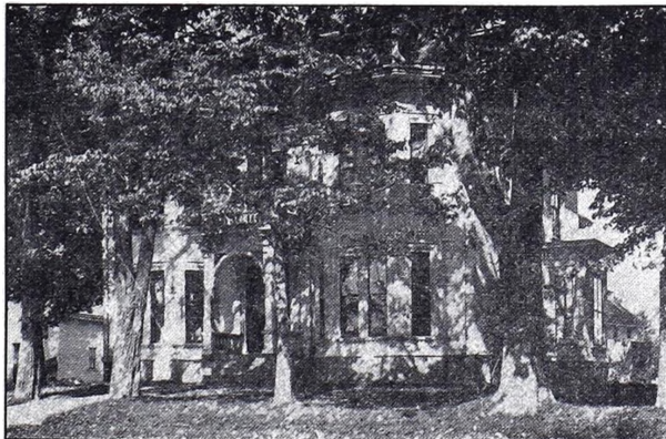
Alpha Tau Omega house used by the fraternity since 1894 was badly damaged by fire
