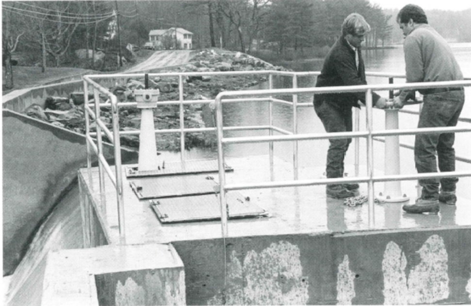
■ Left to right: Gary Stevens, Assistant Plant Operator, and Don Neumann, Foreman, operating the sluice gate.
