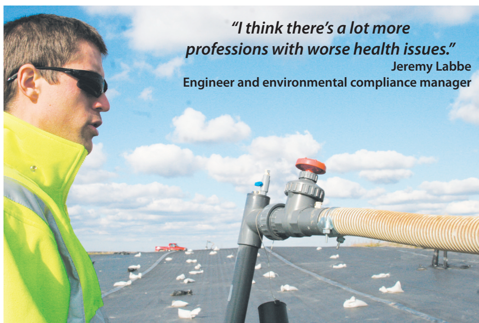
Beth Kevit • News Editor Jeremy Labbe, engineer and environmental compliance manager at Juniper Ridge Landfill, demonstrates the valve system on pipes that draw gas from the landfill.
