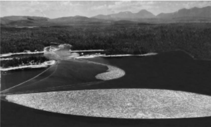
Great Northern Paper Company brought an end to the classic West Branch river drive. The age of steam mechanized much of the log-driving effort with giant boom bags and steam-powered tow boats — the latter converted to diesel by the 1950s when this photo was taken. Courtesy of the Ambajejus Boom House Association.
