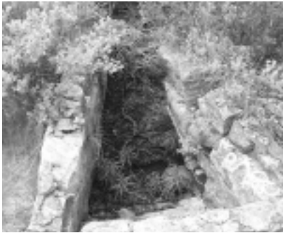
Entrance to cellar with descending stairs.
