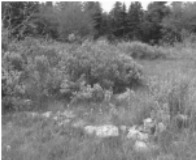
Foundation of back house, connecting the main house and barn.
