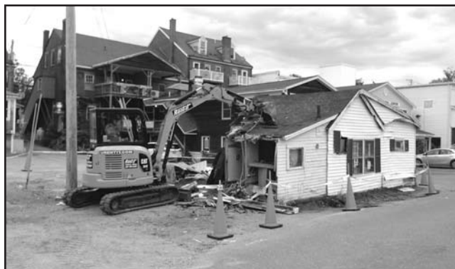
Demolition of the barber shop
