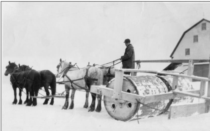
Snow roller, Caribou, 1930. The use of the snow roller was one example of changing ideas about better road maintenance at the end of the nineteenth century. A snow roller was an improvement over a snowplow as it packed down the snow on the roads, creating a wide, hard, smooth surface. Courtesy of the Caribou Public Library, Caribou, Maine.
