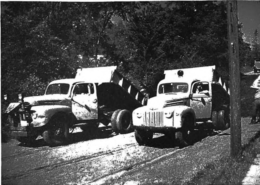
City Trucks spreading tar cover
