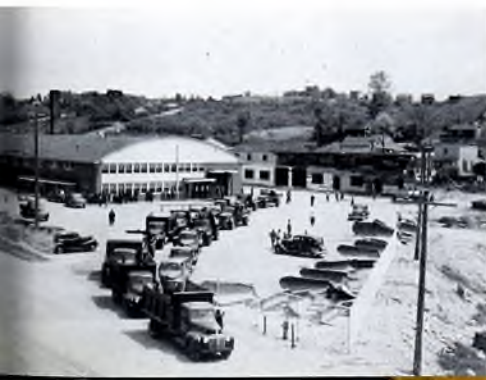
New PWD Building
