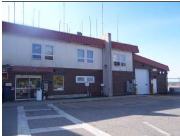
Airport terminal with firefighting addition
