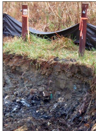
Area 1 remediation removing rubbish from around a water quality monitoring well
