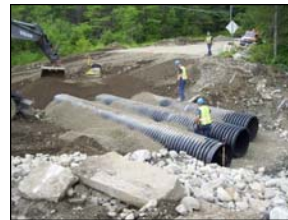
Cony Street culverts replaced
