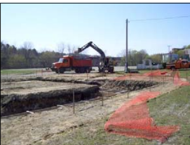
Public Works pavilion work
