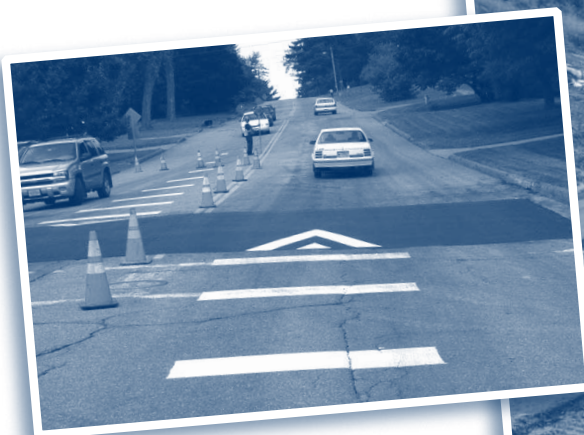
Installing speed table on Winthrop Street
