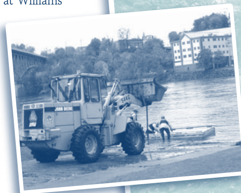
Removing docks from East Side boat landing.
