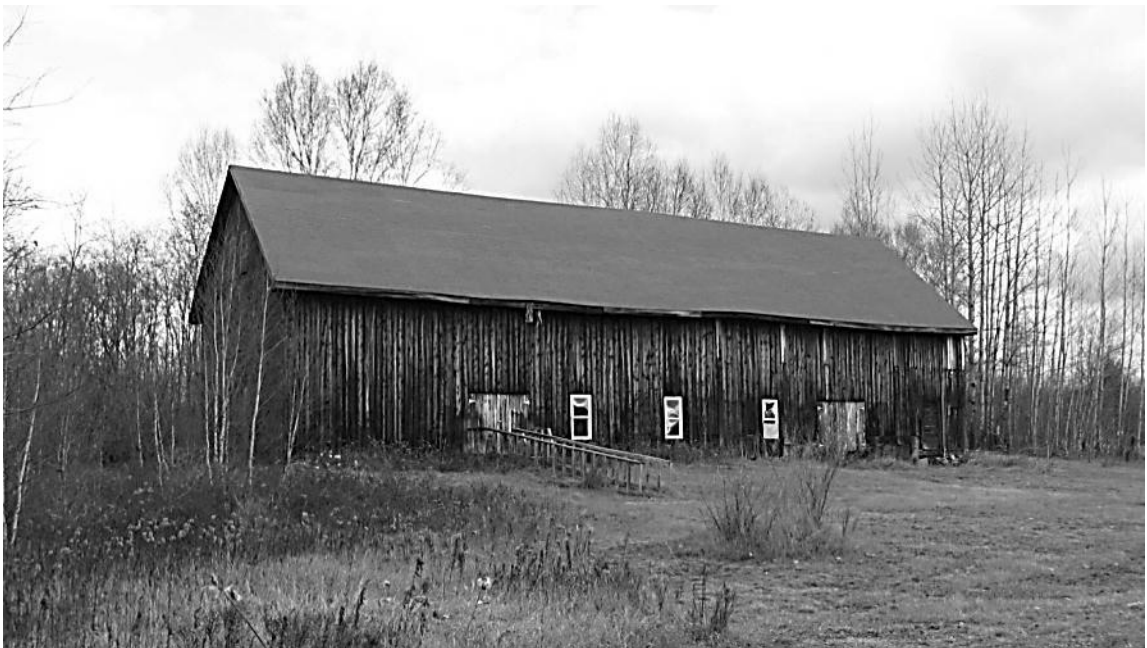
Figure 2: Exterior View of Existing Barn
