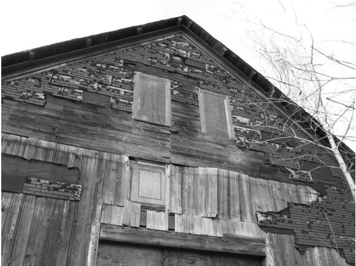
Figure 5: Current Exterior of the Barn
